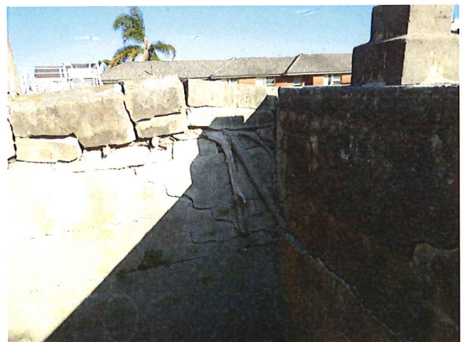
Photo 20 - Cracking to masonry balustrade running up external stair
