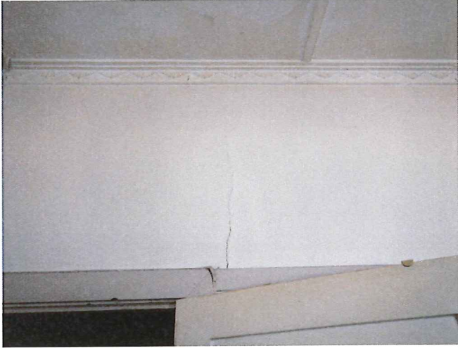
Photo 29 - Evidence of cracking to the internal walls of the upper level apartments
