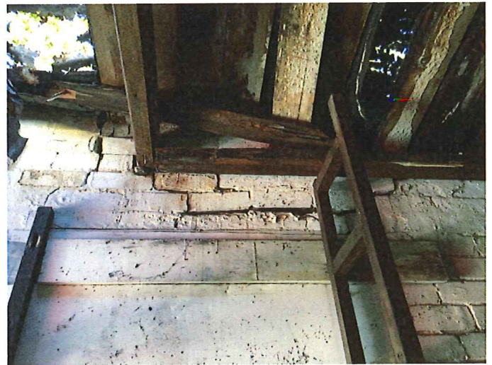
Photo 10 - Damage over window as a result of corroded lintel
