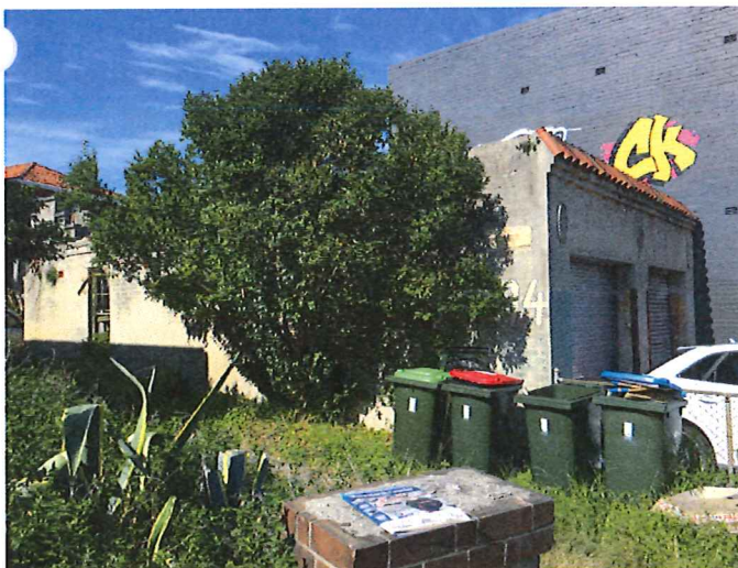
Photo 3 - Existing garage structure
