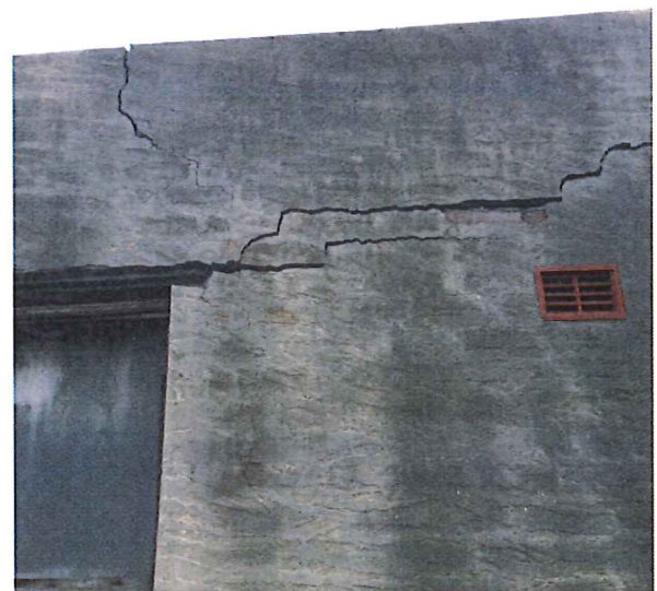
Photo 12 - Damage over window as a result of corroded lintel
