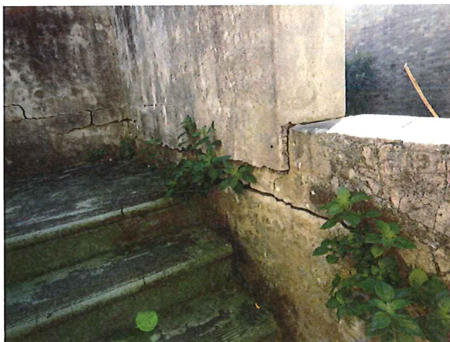
Photo 19 - Cracking to masonry balustrade running up external stair
